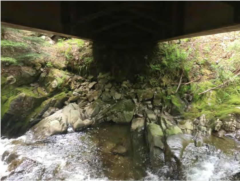
Right Bank Abutment when facing downstream
