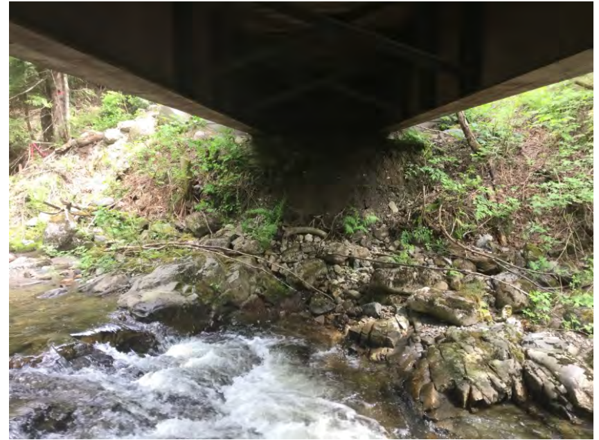
Left Bank Abutment when facing downstream
